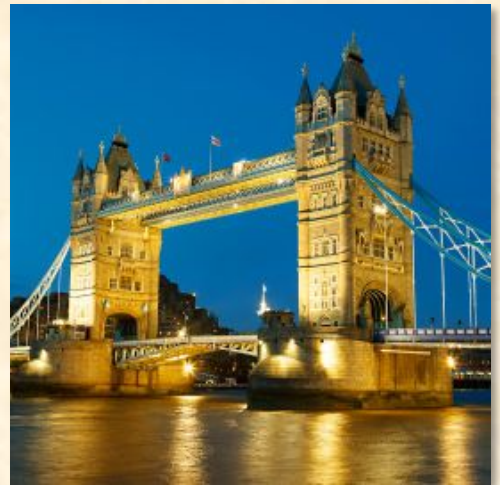
Bridge at night, London
